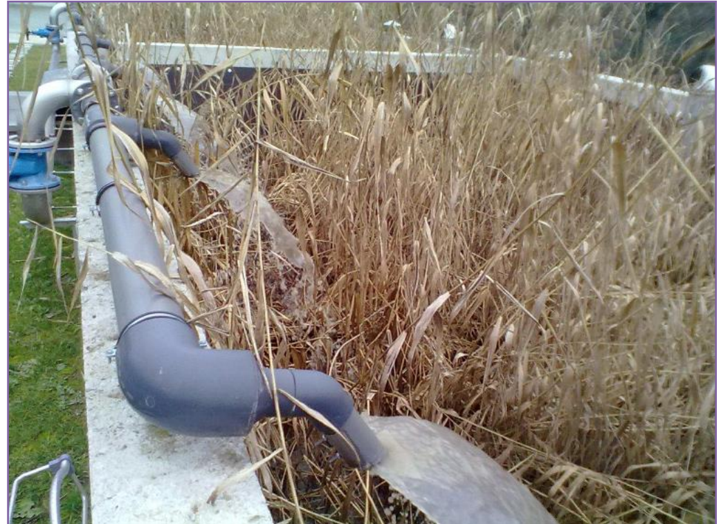
Spreading pipes
