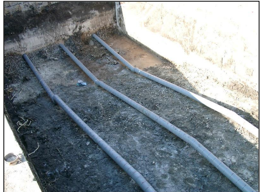
Drainage/aeration pipes
